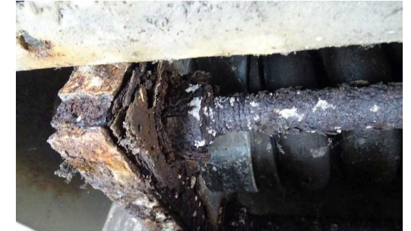
Gallows Corner Flyover (steel fatigue) Daily users – 38,000
