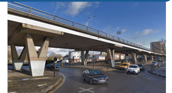
Croydon Flyover (significant structural lighting renewal) Daily users – 40,000
