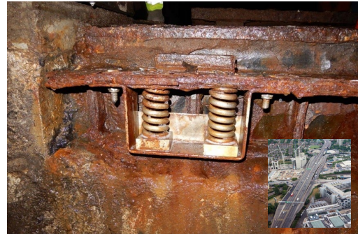
A40 Westway (12 x key bridge Joint renewals) Daily users – 90,000
